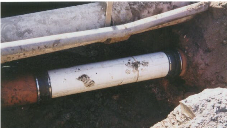
Figure 4. On Marine Drive, 12" sewer pipe repairs completed by Public Works (September 2001) Photo by Jon Walter
